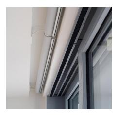
Blinds installed inside a window recess look neat, but you need to factor in light gaps at the side. Ensure you have enough space to accommodate the depth of the blind.
